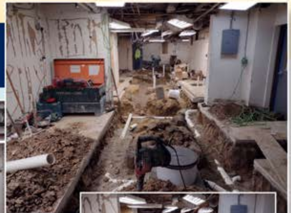
Building of Kitchen Floor
